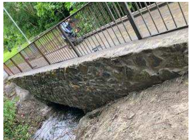
Santry Footbridge repairs and new railings
