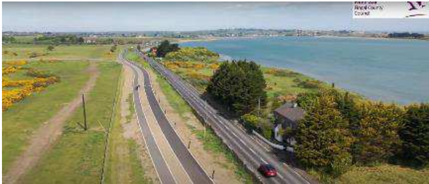
B aldoyle – Portmarnock Greenway - Completed
