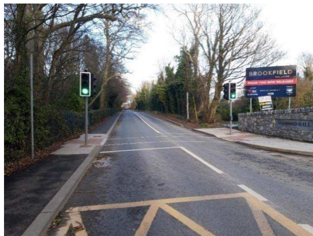
Newly commissioned pedestrian signals on the Back Road Malahide
