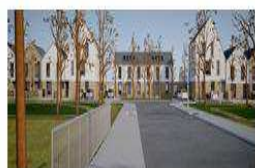
Street view towards north units
