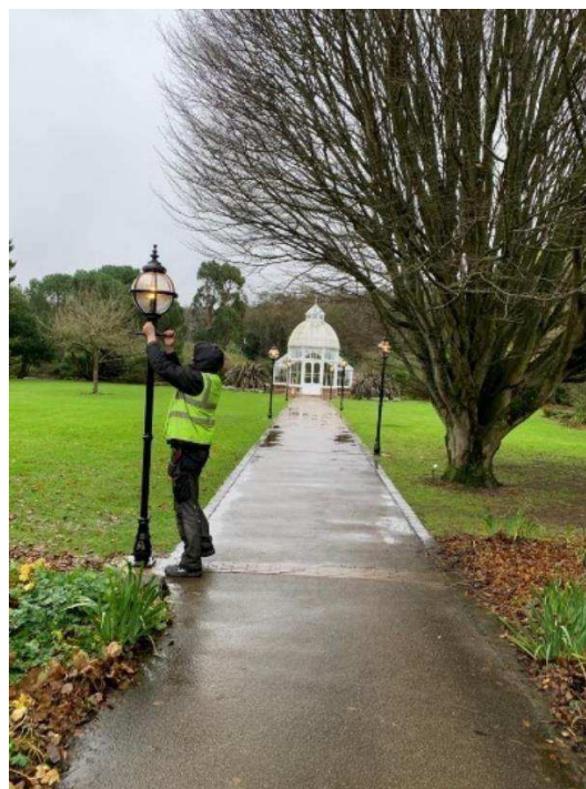
Replacing lights in Malahide Castle Walled Garden
