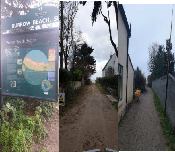
Works carried out at Burrow Beach access routes in preparation for summer 2021
