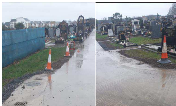
Drainage remediation works carried out at Fingal Burial Ground
