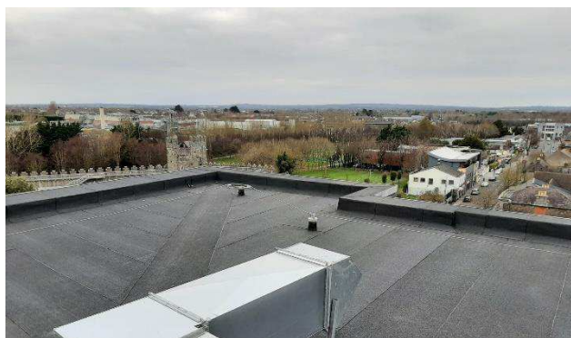
Roof repair works in County Hall
