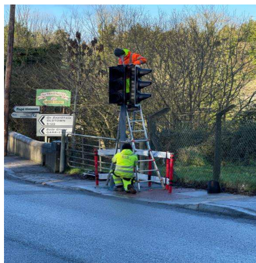
Civil works now complete for the Pedestrian Crossing at Naul GAA ground.
