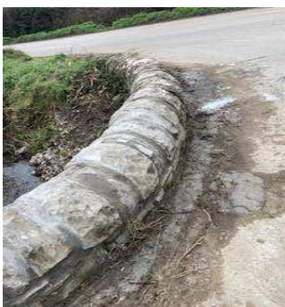
Rowlestown Culvert wall repair
