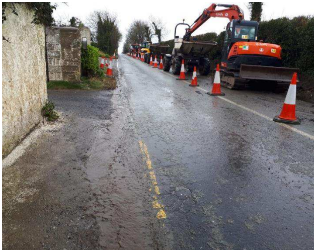
Works on the Foul Sewer Rising Mains progressed onto the R128 Road in Mid-February with works progressing well.
