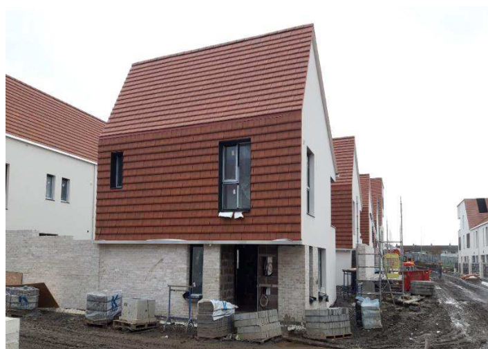
65 units under construction at Ladyswell, Dublin 15
