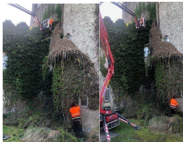
Ivy removal at Malahide Castle to facilitate structural works
